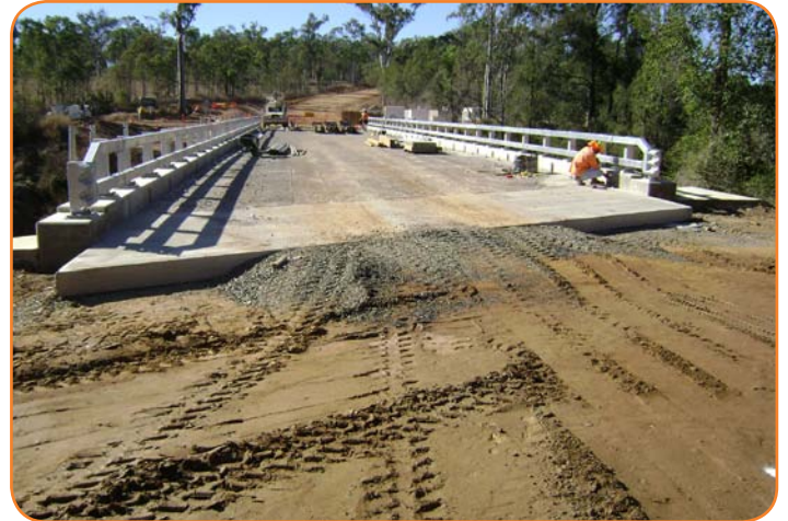
Replacement works continue on Two Mile Creek bridge
